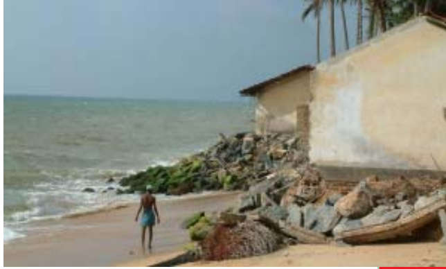
Coastal Erosion in Ulhithiyawa, Wennappuwa, 2003
